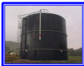
Deerfield Water Storage Tank
