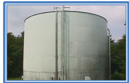
Existing Churchville Water Storage Tank
